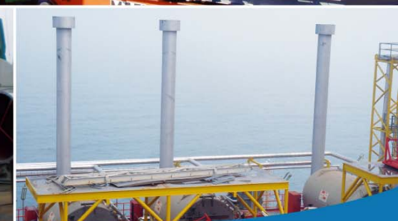
3x5000kW (3x17 MBtu/h) (Gas, diesel oil & crude oil fired) CNOOC Nanbao Offshore Oil Field 中国海洋石油CNOOC 南堡油田 (海上平台)
